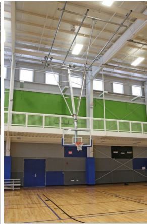
Each ceiling suspended basketball backstop was custom-designed to work within the facility space, while column protective pads were finished in field for a perfect fit.
